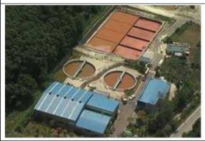
Hambaek mine was operated from 1955 to 1993, during the mining operation, it produced about 17 million tons of anthracite. As acid mine drainage (AMD) from the mine has been a serious problem, both electrochemical and passive treatment system were adopted with the capacity of 7,200 m per day.
