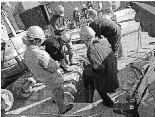
Replacement of service pipe (Module 3)
