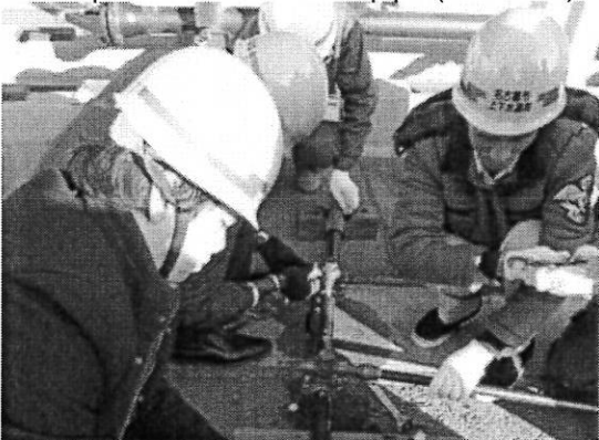
Practical work of service pipe connection (Module 3)
